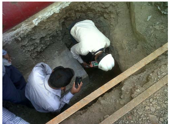
Rebar Mapping of Footing
