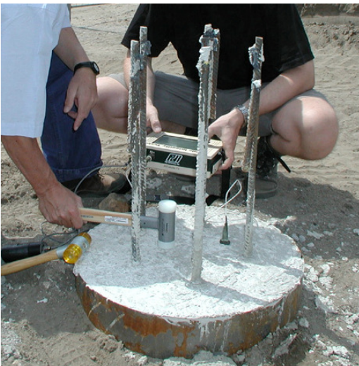
Pile Integrity Test
