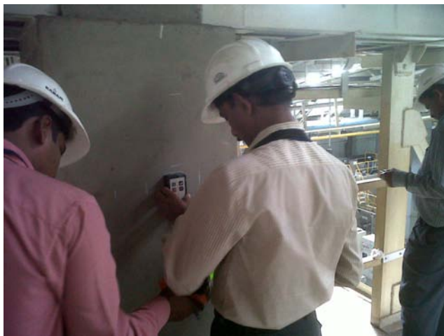
Rebar Mapping of column
