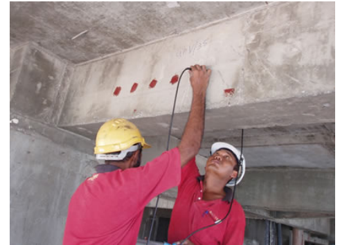
UPV Test on a beam
