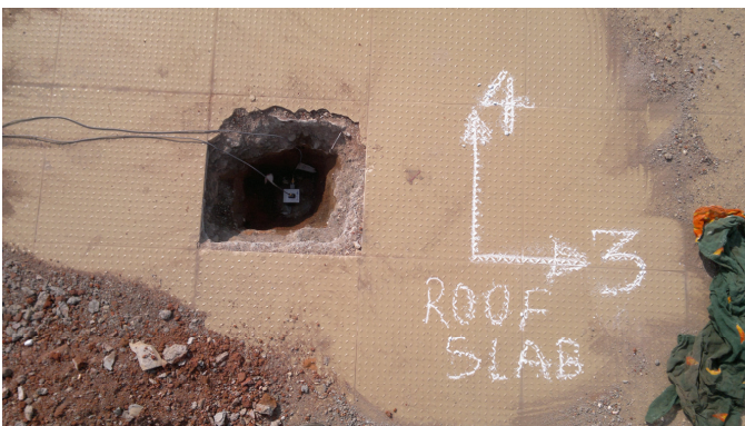
Accelerometer fixed to terrace slab
